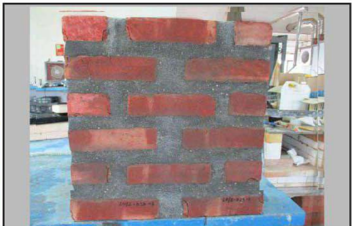
Photograph 2: Image of the panel damage after 100 cycles of Freeze/Thaw (none)
